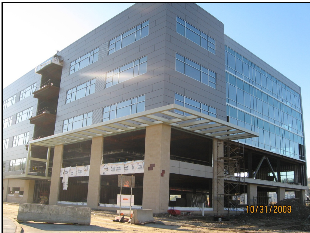
Figure A – October Progress Photo
